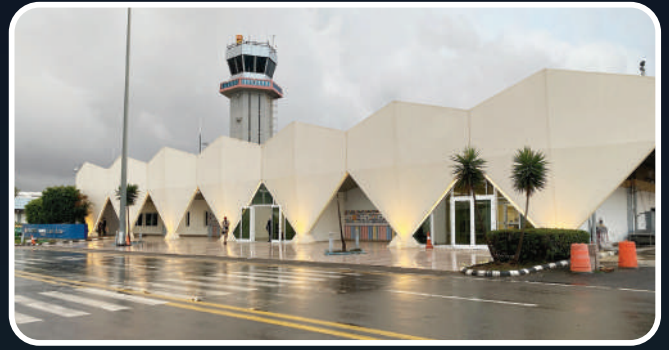
Abha Regional Airport Terminal Expansion
