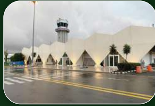
Abha Regional Airport Terminal Expansion
